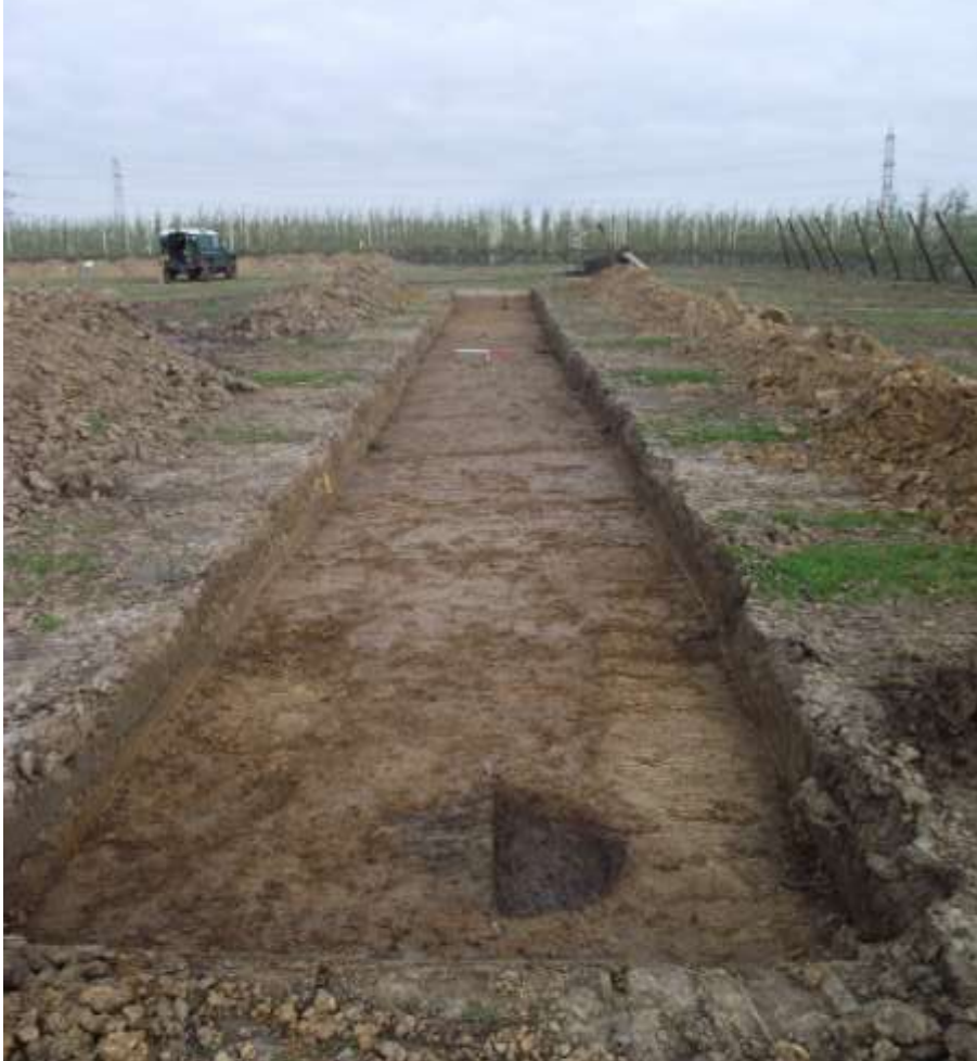
Plate 5 – General shot of Trench 3, looking northwest
